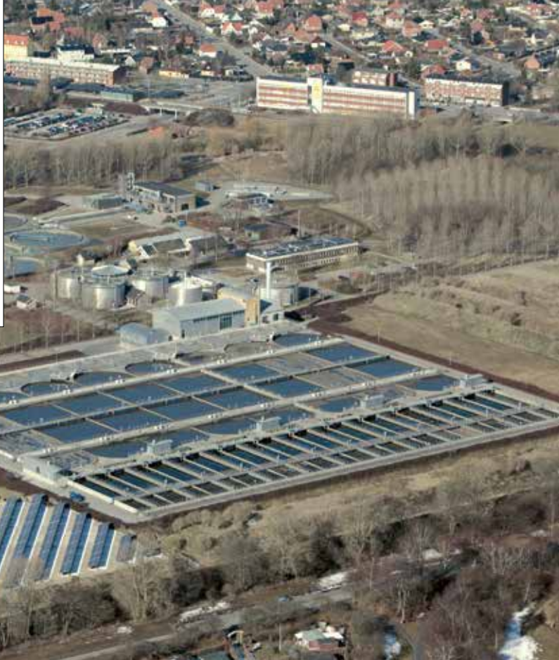
PHOTO VOLTAICS AT DAMHUSAEN IN VALBY, THE LARGEST PHOTO VOLTAIC PLANT IN THE NORDIC COUNTRIES. 8% OF THE ELECTRICITY FOR THE CLEANING OF THE WASTE WATER IS COVERED BY PV. THE PLANT IS OWNED BY "LYNETTE COOPERATIVE" IN COPENHAGEN, AND - SUPPLEMENTED WITH BIOGAS FOR THE PRODUCTION OF ELECTRICITY, THE PLANT COVERS ALMOST 50% OF THE YEARLY CONSUMPTION OF ELECTRICITY
