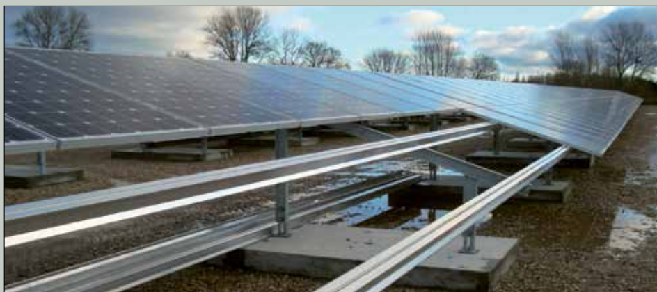
DETAILLE OF THE FUNDAMENT FOR THE PHOTO VOLTAIC
