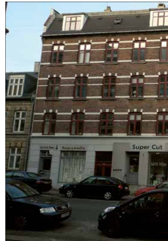
THE HOUSING ESTATE AT GL. JERNBANEVEJ I VALBY – BEFORE THE RETROFITTING
